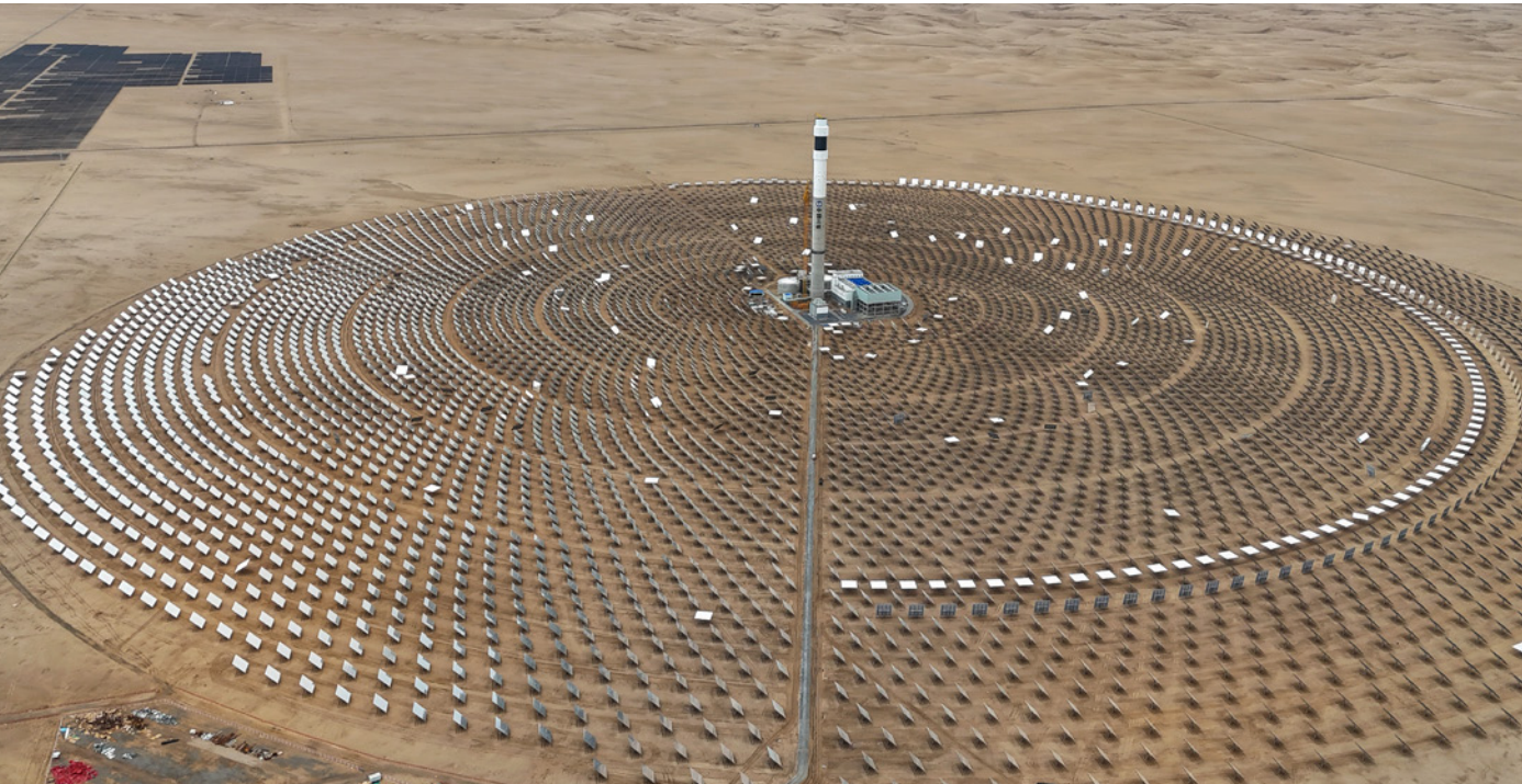
A solar energy molten salt power tower project in the northwest desert of China. By reflecting sunlight through about 2,000 mirrors and melting the salt at the top of the tower to generate electricity, an Alimak SL500 industrial lift was installed inside the tower.
