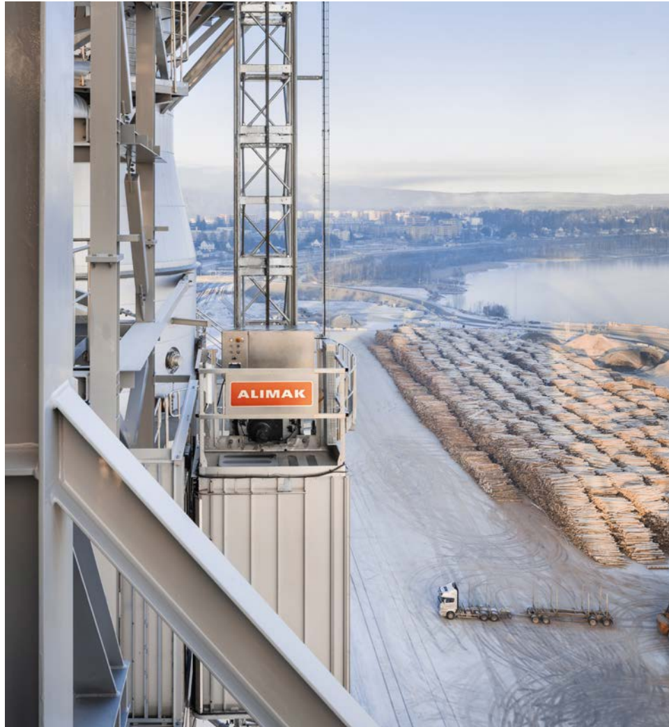
An Alimak industrial elevator at the world's largest production line for bleached softwood kraft pulp – the Östrand pulp mill in Timrå, Sweden.
