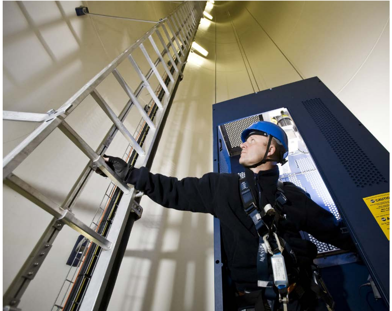
Safe service work inside a wind turbine.
